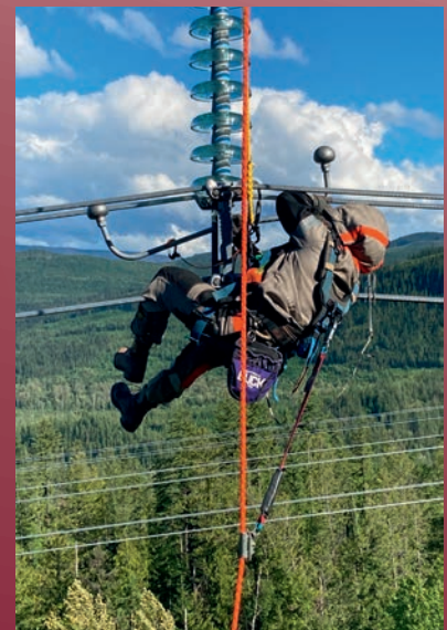
A Local 258 Power Line Technician performing barehand work in Vernon, BC.
